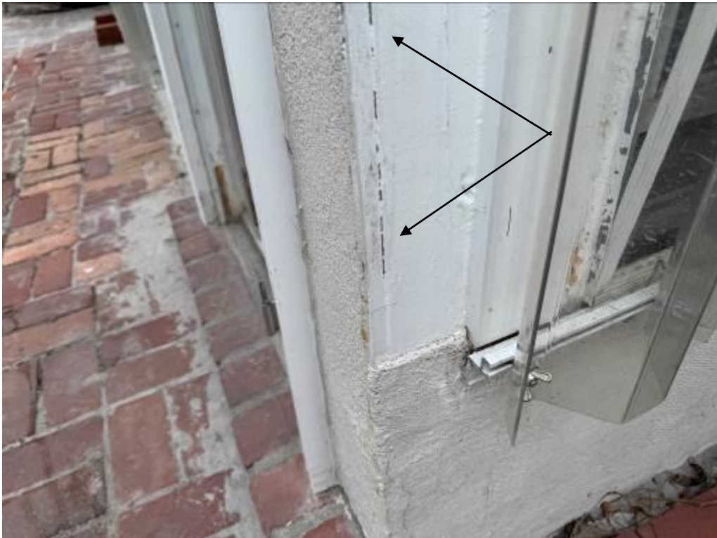
Photo No. 10: Reported cracking/separation at rear patio column/support framing.
