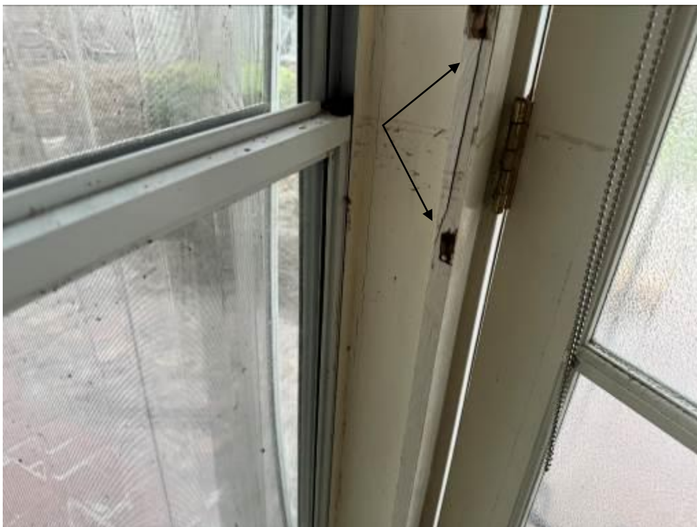
Photo No. 8: Cracked door frame in rear enclosed patio.
