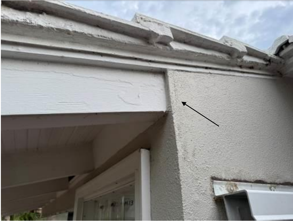
Photo No. 9: Stucco cracking along rear roof overhang.
