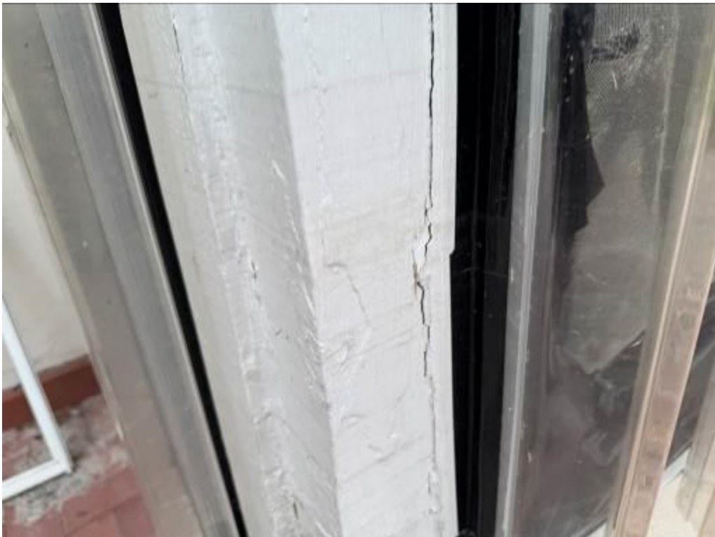
Photo No. 12: Cracking/separation of rear patio framing.
